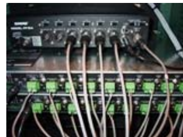
Laying out the I/O wiring.
